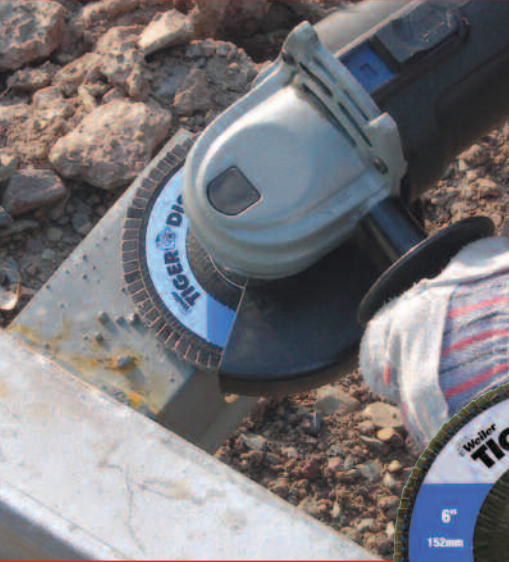
Removing heavy weld spatter while prepping surface for painting.
